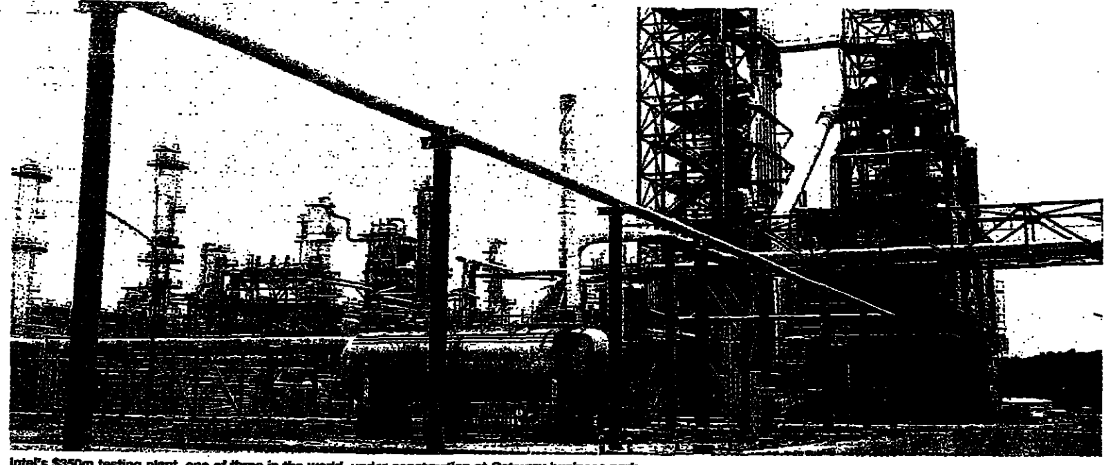
Intel's $350m testing plant, one of three in the world, under construction at Gateway business park.
